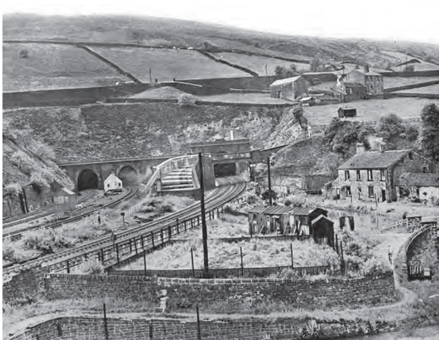
Looking southwest towards the Marsden end of Standedge Tunnel. The single-track 1871 (left) and 1848 (right) railway tunnels are on the left with the 1893 twin-track tunnel to their right. Between the tunnels, the overflow from the Tunnel End Reservoir is seen. The canal tunnel was extended by 11 yards in 1822 when the overflow was diverted over the tunnel mouth. The tunnel mouth with a bridge across it is seen to the left of Tunnel End cottages. Tunnel End Footbridge No 62 is on the right with part of Tunnel End Winding Hole in the foreground
